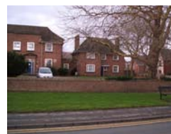
Protected trees on edge of site
